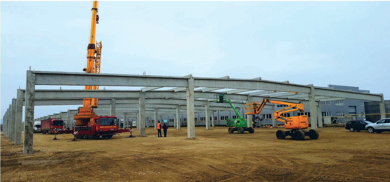
Hala Barrier - BACĂU
